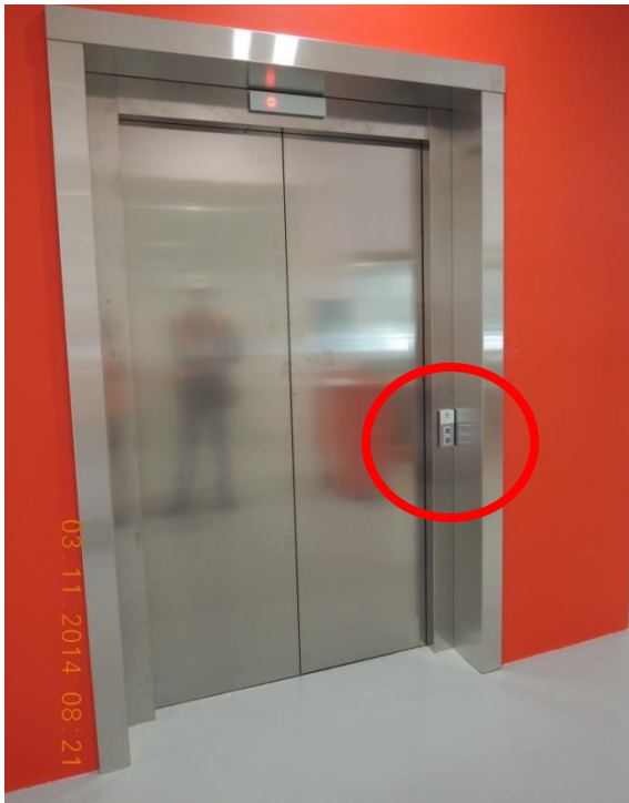
Figure 5 image of non-compliant lift call button installation
